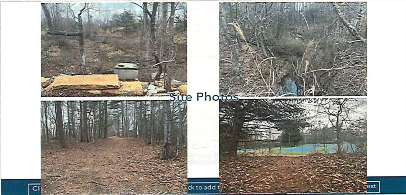
1 – Going back to the culvert in the drive, this photo is facing north looking at an existing stormwater detention basin. This flows under the driveway 2 – if you did a 180 on top of the culvert to face south, you see an open stream that originates here. This stream collects the stormwater from the Michelle Dr and the developments accessed off of it. If flows south and feeds a pond on the Camp Pinewood Property. 3 – This is a photo of Sarasota Ln at the south end of the property. This is a cleared but unpaved ROW. There is public sewer located in this ROW. 4 – Across Sarasota Ln to the south you can see the neighboring amenities at Camp Pinewood
