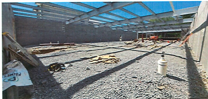
Biosolids Thermal Dryer Facility Construction. April 2026.
