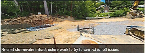
Recent stormwater infrastructure work to try to correct runoff issues
