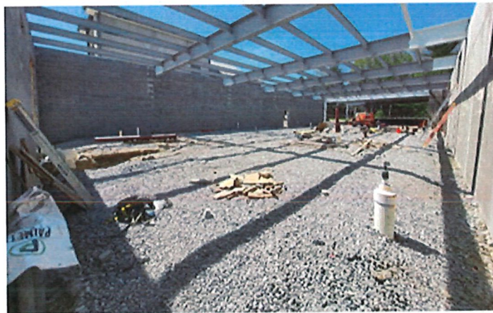
Biosolids Thermal Dryer Facility Construction. April 2026.
